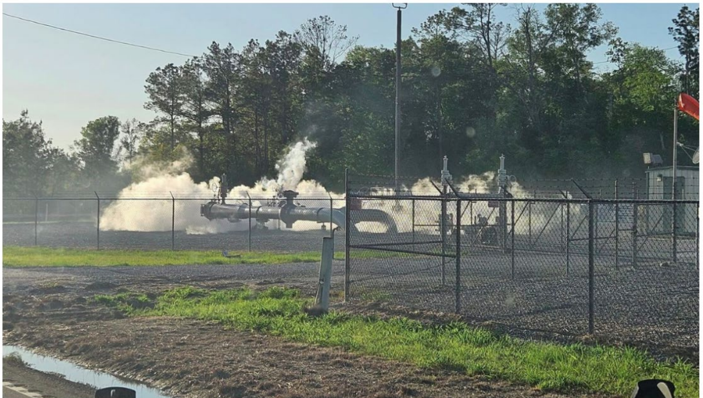
☑ Clouds of water vapor and carbon dioxide gas escape from a CO2 pipeline near Sulphur in southwest Louisiana on April 3, 2024. The harmful gas prompted a shelter-in-place advisory and concerns about pipeline safety and warning systems. (Photo courtesy of Ward 6 Fire Protection District)
