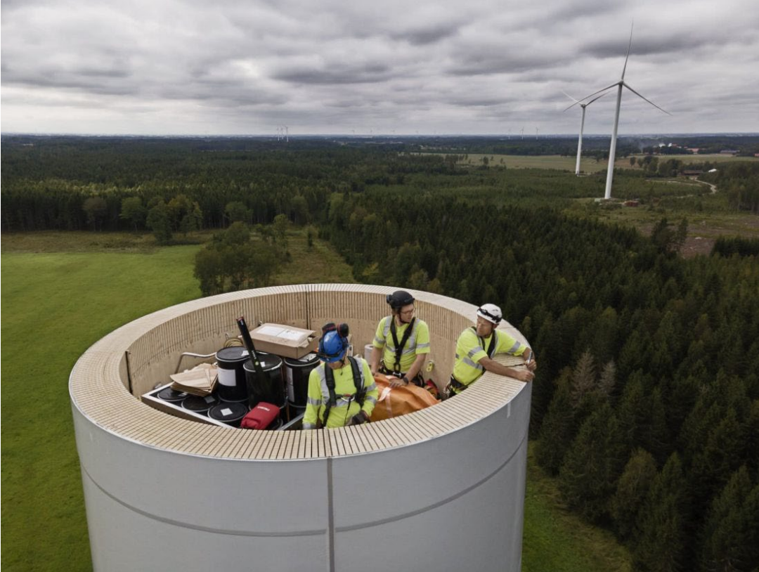
Assembling the wooden tower modules on site. Paul Wennerholm/Modvion
