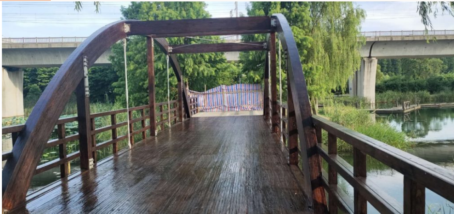
Renovated timber bridge
