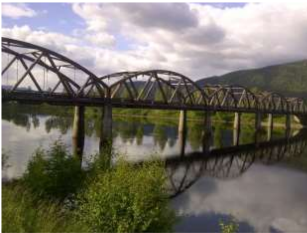
Figure 4-32: Evenstad Bridge is made up of five glulam truss spans, each 36m (118ft) long. The trusses support steel cross beams and a stress-laminated deck.
