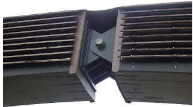
Figure 4-30: Skogsrud Bridge in Tangen, Norway consists of two glulam arches and a stress-laminated deck. The arches are protected with metal flashing on top and wood louvers on the vertical faces. This shelters the elements from rain while still allowing sufficient air flow to keep the moisture content of the wood low.
