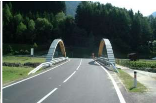
Figure 4-36: Krystalbrücke consists of two glulam tied-arches. These support steel hangers which carry the transverse glulam beams which, in turn, carry the deck. This bridge has been in service since 1995.
