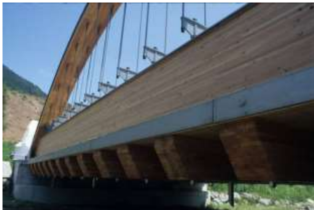
Figure 4-36: Krystalbrücke consists of two glulam tied-arches. These support steel hangers which carry the transverse glulam beams which, in turn, carry the deck. This bridge has been in service since 1995.
