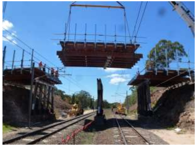
Figure 4-40: Boundary Road Bridge is a four-span overpass crossing a pair of Queensland Rail tracks. The light weight of the timber superstructure allowed each span to be preassembled alongside the road and lifted into place by crane. This limited the interruptions to rail traffic on the tracks below. This bridge was installed in 41 hours.
