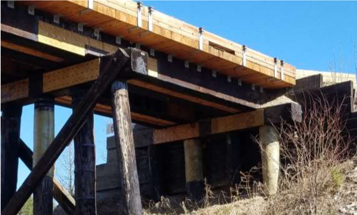
Figure 4-19: The Existing piles, caps, and chords were reinforced with high-strength fiber to restore capacity that had been lost due to decay. The old deck was removed and replaced with a new transverse glulam timber deck and curb.
