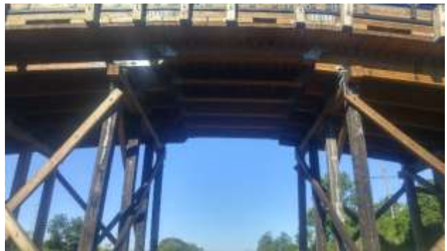
Figure 4-22: Dickinson Road Bridge, in Port Hope, Ontario consists of six glulam girder lines. The substructure was completely rebuilt; however, much of the material from the original structure was salvaged for use in the new bridge.
