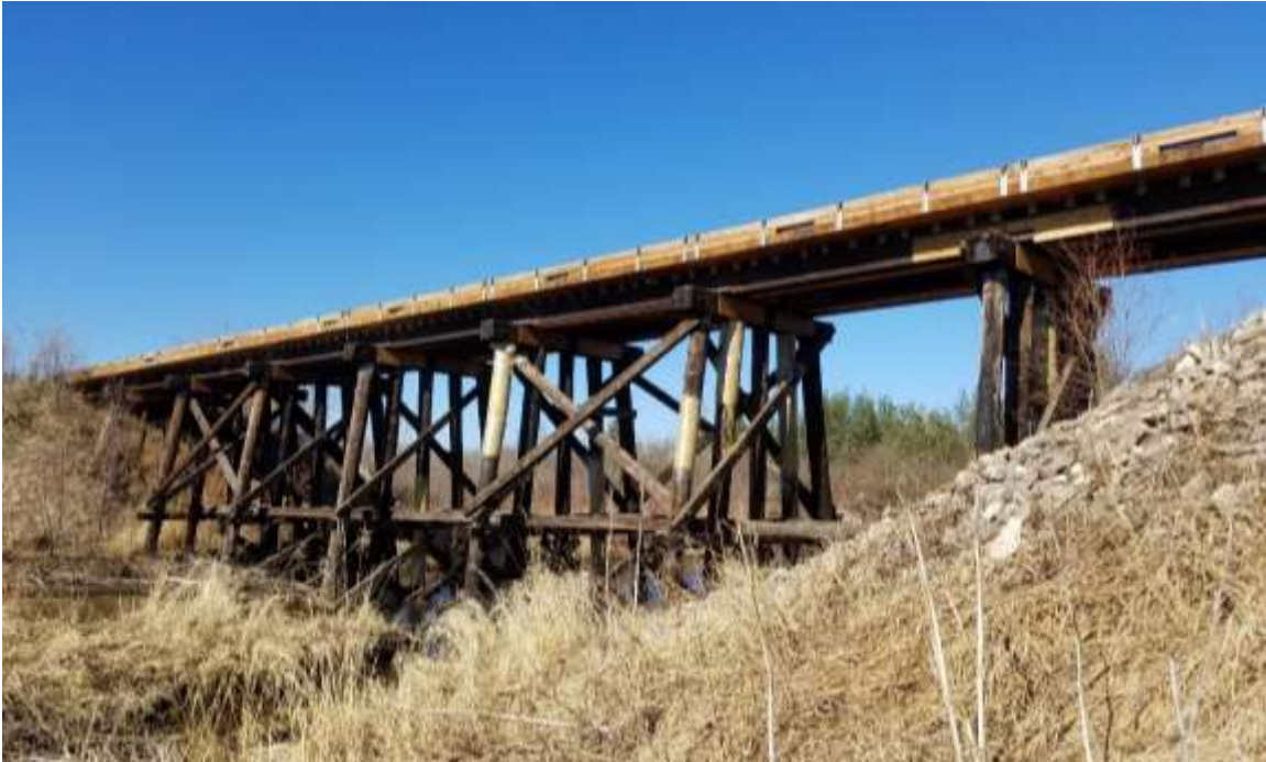
Figure 4-18: Meadow Lake Bridge is a conversion of a decommissioned railroad trestle to be used as a forestry bridge.
