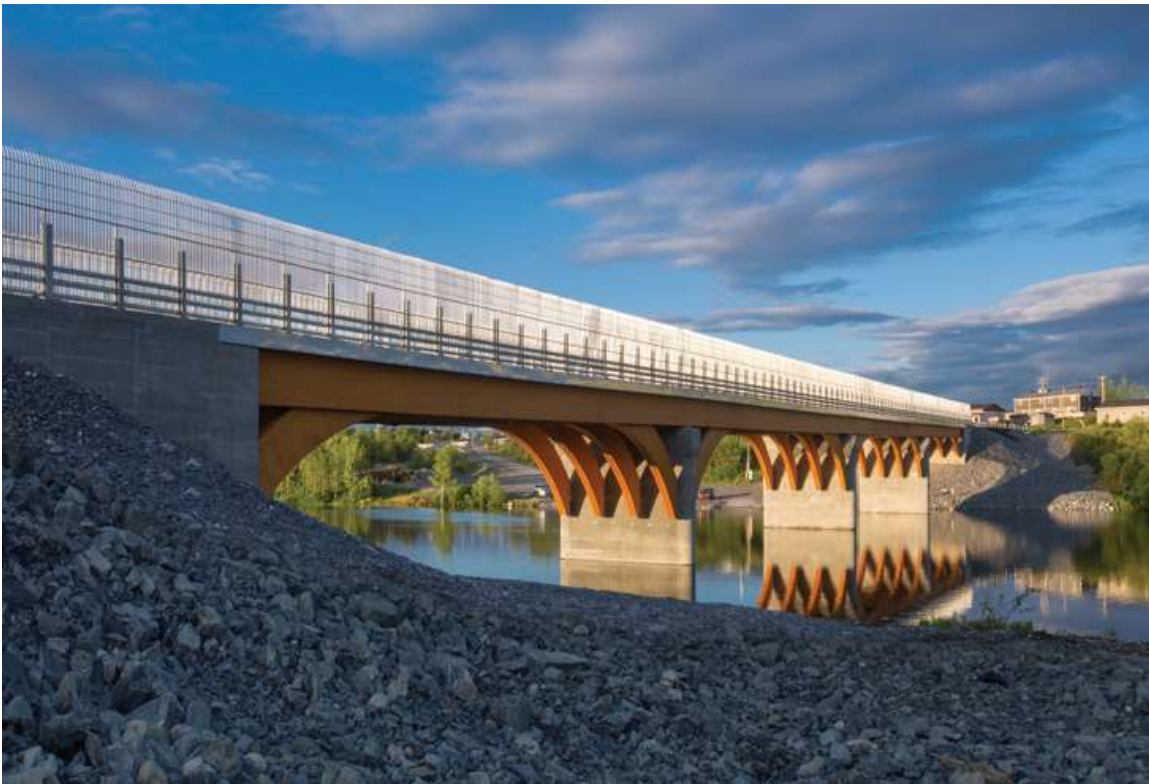
Figure 4-24: Mistissini Bridge is a 4-span bridge totaling 160m (525ft) long. The bridge is 9.25m (30ft) carrying two lanes of traffic, plus a pedestrian walkway on one side. It consists of glulam girders and arched knee-braces supporting a glulam deck with an asphalt wear-surface. (Forestric Nordic, 2015)
