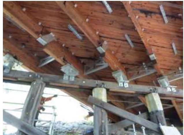
Figure 4-39: Alderley Avenue Bridge crosses a pair of Queensland Rail tracks. The new glulam superstructure and deck were installed on the existing substructure. Localized decay in the substructure was repaired using high-strength fiber wraps on the piles and tension reinforcement on the headstocks. This bridge was installed in 39.5 hours. From the start of design phase to the completion of works was 65 days.
