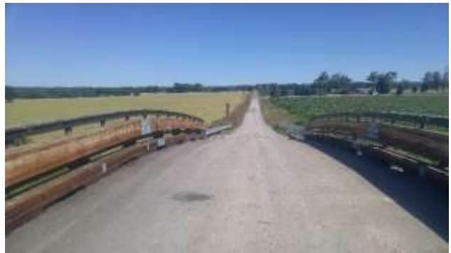
Figure 4-20: Providence Road Bridge in Clarington, Ontario consists of five lines of glulam girders supporting a transverse timber deck. The existing solid sawn frame bents were restored, including the addition of high-strength fiber reinforcing in some locations to restore capacity that had been lost due to decay. An asphalt wear surface was installed on top of the transverse timber deck. The timber guard rail is crash-tested to TL-4 specifications.
