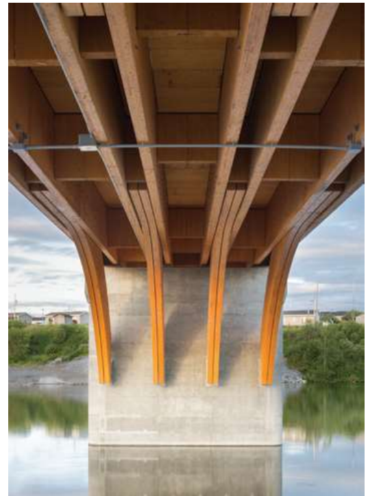
Figure 4-25: The arched braces are connected to the piers with pinned connections. The connection between the arches and the girders serves to both support the girder ends and to create a moment-resisting splice in the girders. This forms a continuous structure with no deck joints, which will help avoid cracking of the asphalt and maintain a waterproof surface. (Forestric Nordic, 2015)
