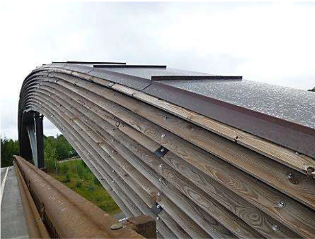
Figure 4-30: Skogsrud Bridge in Tangen, Norway consists of two glulam arches and a stress-laminated deck. The arches are protected with metal flashing on top and wood louvers on the vertical faces. This shelters the elements from rain while still allowing sufficient air flow to keep the moisture content of the wood low.
