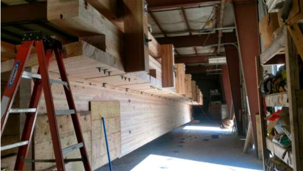
Figure 4-17: All timber components are fabricated and pre-assembled in the shop prior to preservative treatment. This dry-fit process helps avoid any field modifications that might compromise the preservative treatment layer. The bridge is then disassembled and the components are pressure-treated. They will later be shipped to the site for final assembly. The bridge incorporates an all timber TL4 truck crash proof rail system. The abutments are totally constructed of wood as well. The use of timber abutments versus concrete allows a much shorter construction period as there are no cure time issues relating to placement of the superstructure.
