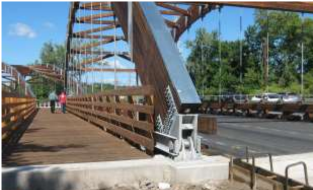
Figure 4-23: Overpeck Park Bridges, by Western Wood Structures, are a pair of two identical through-arch bridges. Each bridge spans 43m (140ft) and carries two lanes of traffic and a pedestrian walkway. The arches are three-pin arches, with a hinge at mid-span; to reduce the size of the individual members, each arch segment is broken into two pieces with a moment splice at its midpoint.
