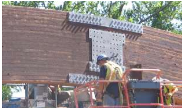
Figure 4-23: Overpeck Park Bridges, by Western Wood Structures, are a pair of two identical through-arch bridges. Each bridge spans 43m (140ft) and carries two lanes of traffic and a pedestrian walkway. The arches are three-pin arches, with a hinge at mid-span; to reduce the size of the individual members, each arch segment is broken into two pieces with a moment splice at its midpoint.
