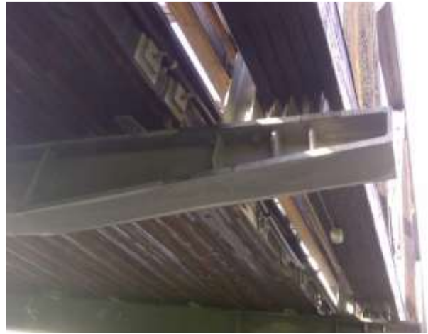
Figure 4-32: Evenstad Bridge is made up of five glulam truss spans, each 36m (118ft) long. The trusses support steel cross beams and a stress-laminated deck.
