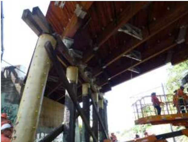
Figure 4-39: Alderley Avenue Bridge crosses a pair of Queensland Rail tracks. The new glulam superstructure and deck were installed on the existing substructure. Localized decay in the substructure was repaired using high-strength fiber wraps on the piles and tension reinforcement on the headstocks. This bridge was installed in 39.5 hours. From the start of design phase to the completion of works was 65 days.
