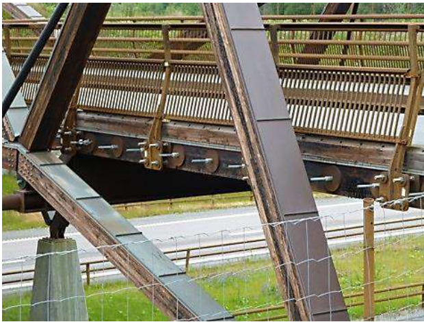
Figure 4-29: Sletta Bridge in Eidsvoll, Norway. The structure consists of asymmetrical glulam trusses which carry steel crossbeams and a stress laminated deck. In addition to being dual preservative treated (with a copper-based preservative and creosote) the main elements are sheltered from moisture using metal flashing.
