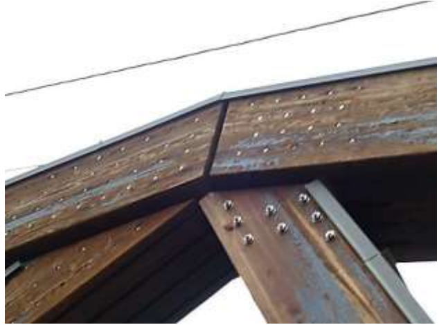
Figure 4-29: Sletta Bridge in Eidsvoll, Norway. The structure consists of asymmetrical glulam trusses which carry steel crossbeams and a stress laminated deck. In addition to being dual preservative treated (with a copper-based preservative and creosote) the main elements are sheltered from moisture using metal flashing.
