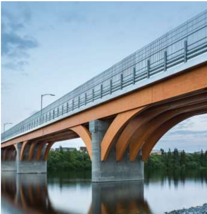
Figure 4-25: The arched braces are connected to the piers with pinned connections. The connection between the arches and the girders serves to both support the girder ends and to create a moment-resisting splice in the girders. This forms a continuous structure with no deck joints, which will help avoid cracking of the asphalt and maintain a waterproof surface. (Forestric Nordic, 2015)
