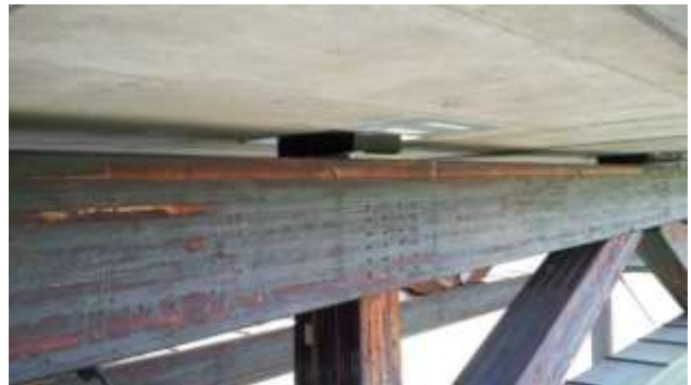
Figure 4-33: Kjølås Bridge consists of a continuous glulam truss with a total length of 145m (476ft) and a maximum span of 36m (118ft). The glulam truss supports a concrete slab deck.
