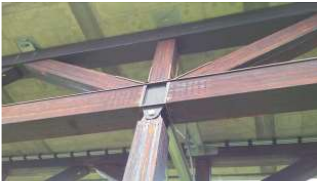
Figure 4-33: Kjølås Bridge consists of a continuous glulam truss with a total length of 145m (476ft) and a maximum span of 36m (118ft). The glulam truss supports a concrete slab deck.
