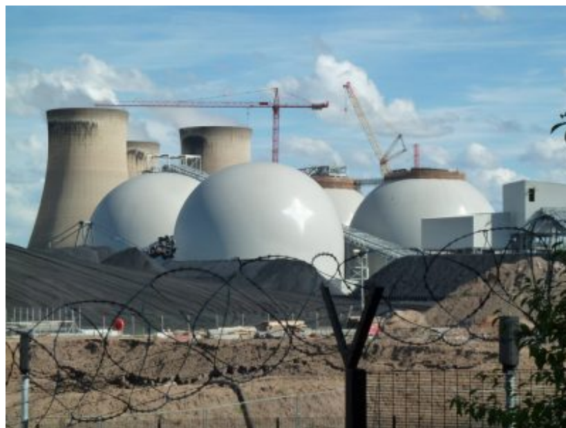
Drax Power Station in North Yorkshire, Great Britain, features inflated storage domes for wood pellet storage as part of a conversion project to mostly biomass firing. Photo: Chris Allen
