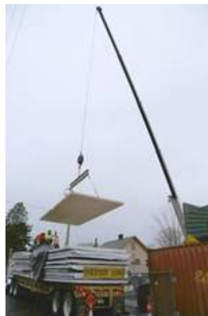
Mass timber is defined by products that are engineered and consist of smaller pieces and are assembled into larger pieces. (WoodWorks photo)
