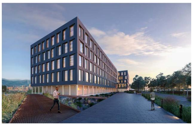
The 150,000-square-foot Catalyst Building in Spokane, Washington, will be the state's first office building constructed of cross-laminated timber. It will also be connected to an energy resource sharing "eco-district" planned for the development.
