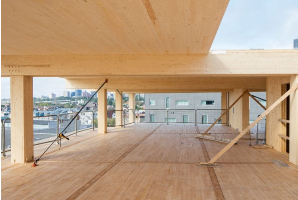
Construction using CLT at the Arbora Complex in Montreal, Quebec. Source: Nordic Structures
