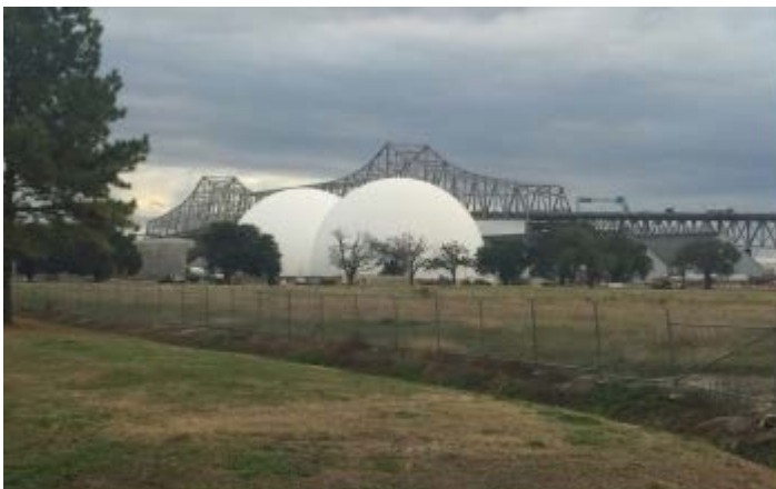
Domes outside Baton Rouge, La., where wood pellets are stored before being shipped to European biomass power plants. Peter Moskowitz/Al Jazeera America
