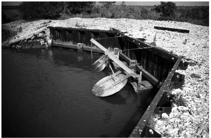
Figure 2. Flap-gated culverts with variable-crest weirs in the spoil banks that separate managed marsh units from canals. The managed units lack levees, allowing water entry into the units during periods of higher water associated with occasional normal tides and frequent winter and tropical storms. Photo courtesy of Joy Merino
