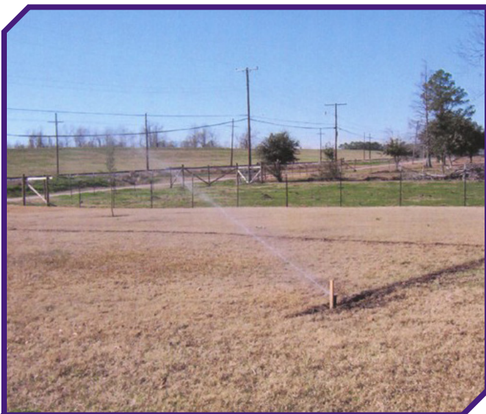
Spray irrigation heads for wastewater effluent. Photo by Richard Grabert
