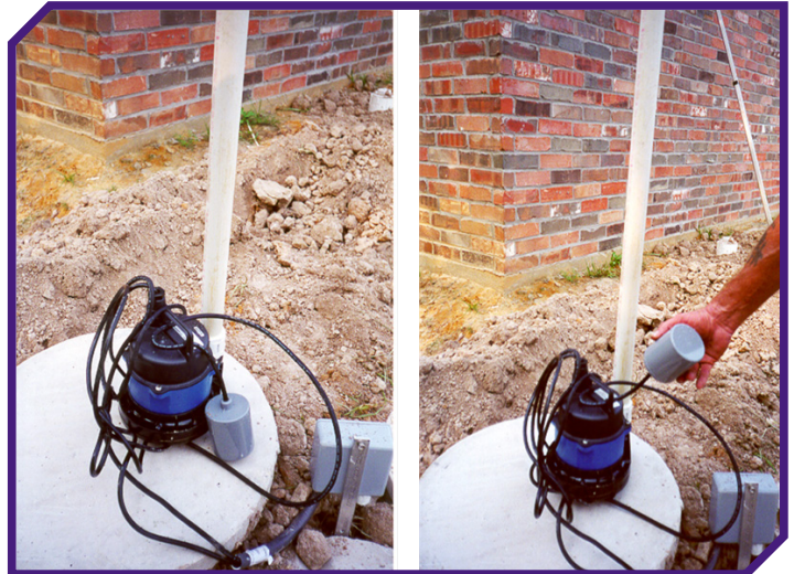
Pumping station installation for septic system. Photo by Richard Grabert.
