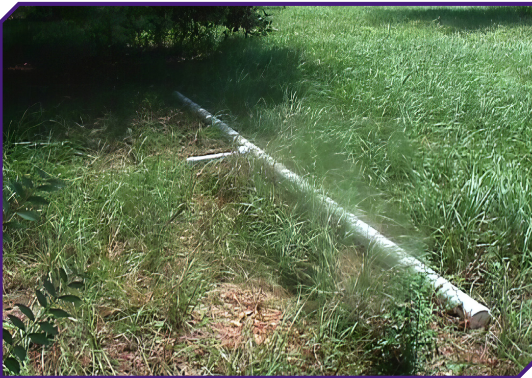
Example image of piping for overland flow. Photo by Richard Grabert
