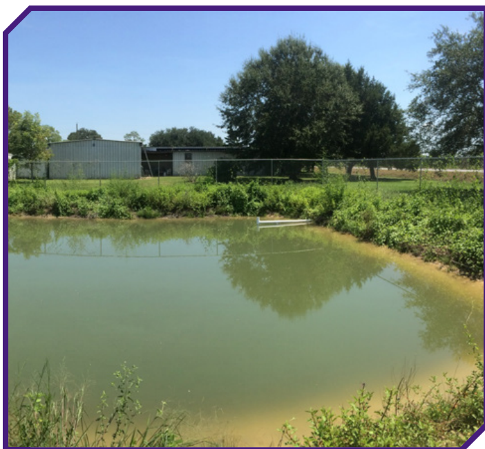
Residential oxidation pond for wastewater effluent. Photo by Richard Grabert
