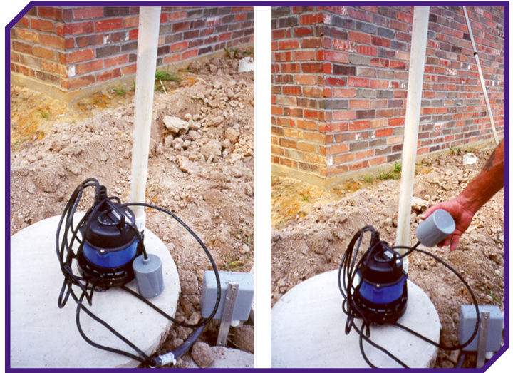
Pumping station installation for septic system. Photo by Richard Grabert.
