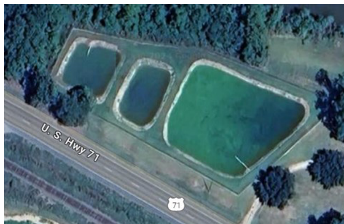
Oxidation ponds are used to treat sewage. Google maps photo
