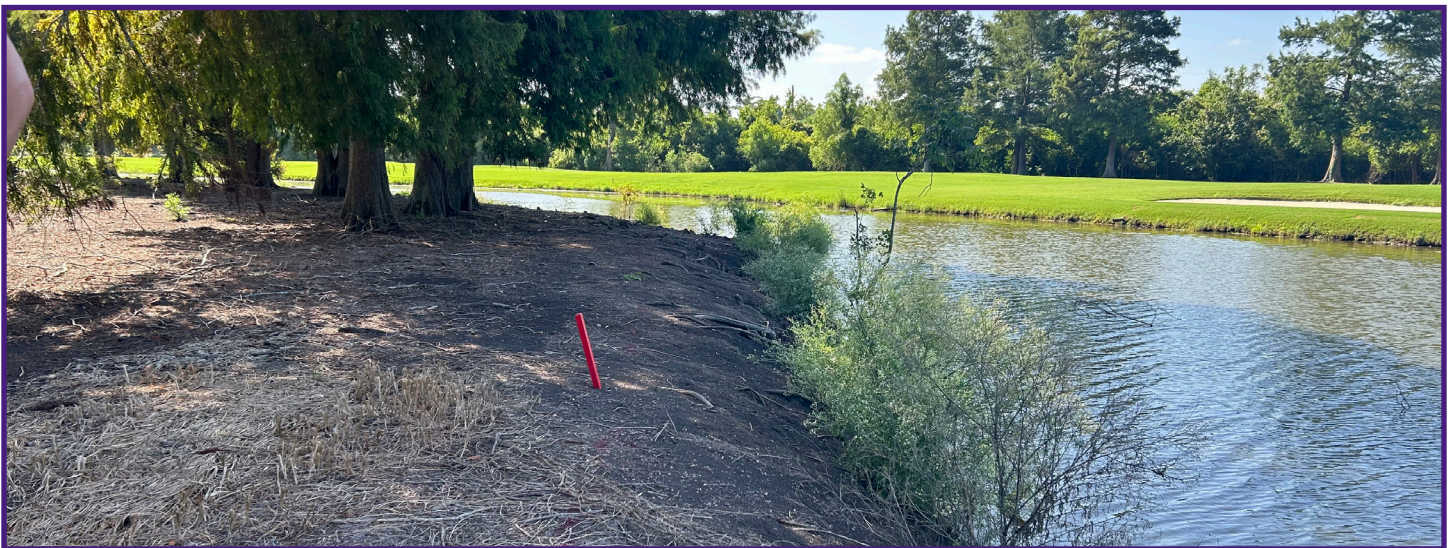
Areas with sloped banks and exposed soil can increase the nutrient or sediment concentration in ponds around the course. Photo by M.P. Hayes
