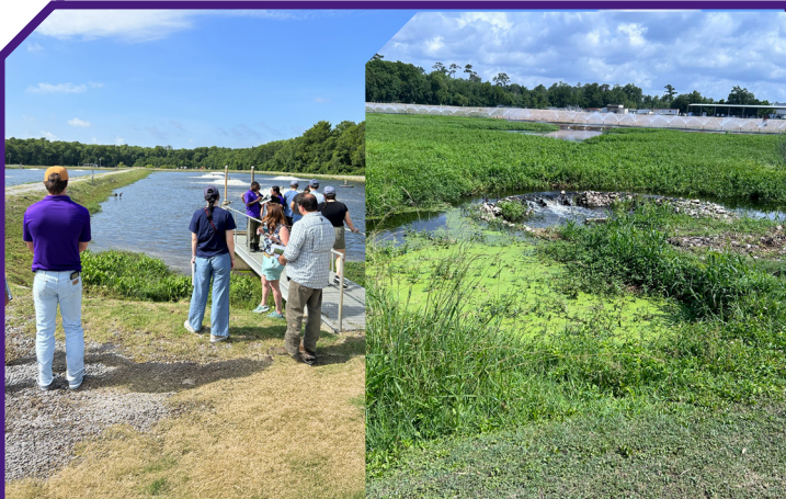
Chemical dosing and treatment efficiency can reduce utilities at wastewater facilities. Photo by LSU ITAC students
